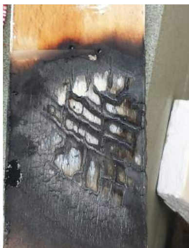
Unprotected wood burns in just a few seconds
